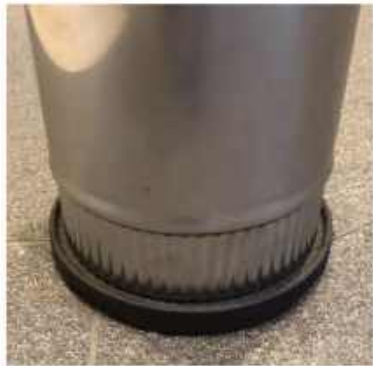
Flue seated correctly.
